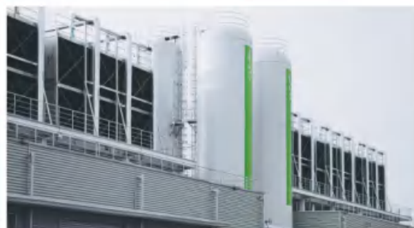
GLP Changshu Cloud Computing R&D and Data Exchange Center, Changshu, Jiangsu (Pinduoduo)
