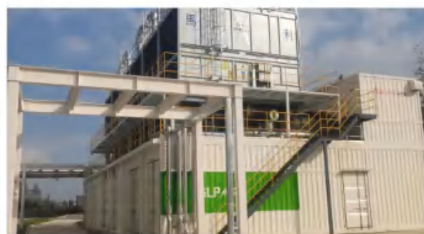
GLP Changshu Cloud Computing R&D and Data Exchange Center, Changshu, Jiangsu (Kingsoft Cloud)
