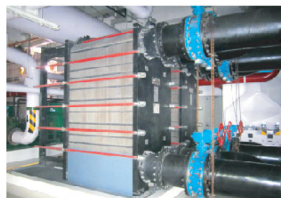
内蒙古酸刺沟电厂/闭式水冷却器/AN40L3 Inner Mongolia Suan-ci-gou electricity generating station
